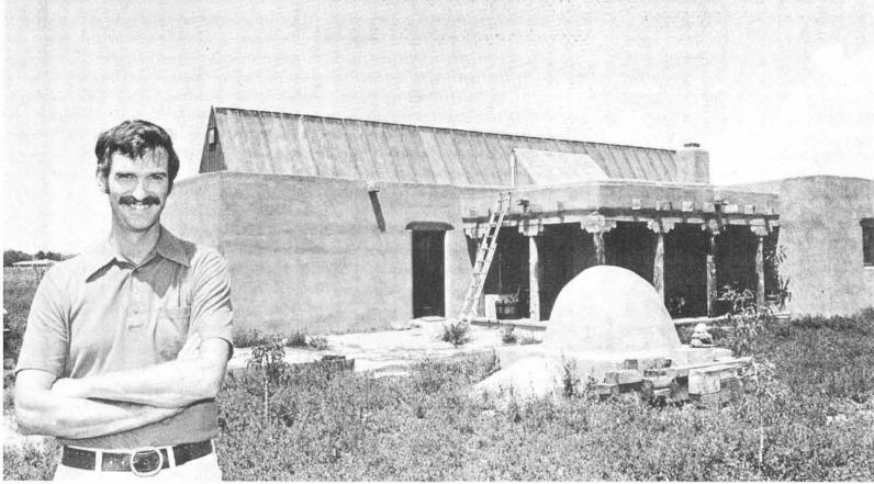
MIKE EDENBURN (5716) at his new adobe home in Peralta. Note large solar collector structure on roof for space heating and smaller collectors for hot water heating.
